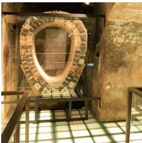
Figure 5-14 – Tank Stream – A salvaged section of brick oviform conduit on display in the former GPO building.
