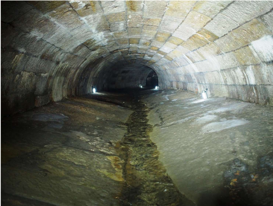
Figure 6-32 – The sandstone masonry arch section of the Tank Stream. Source: Sydney Water
